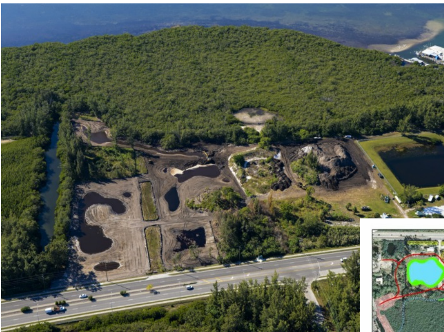
Left: December 2014 aerial of 93 acre FISH Preserve Restoration Project. Project done in partnership with Sarasota Bay Estuary Program, the Southwest Florida Water Management District and Manatee County Government. The first of two phases this project provides a substantial beginning to the 98 acre restoration. Below: Full Conceptual Restoration Plan for the FISH Preserve.
